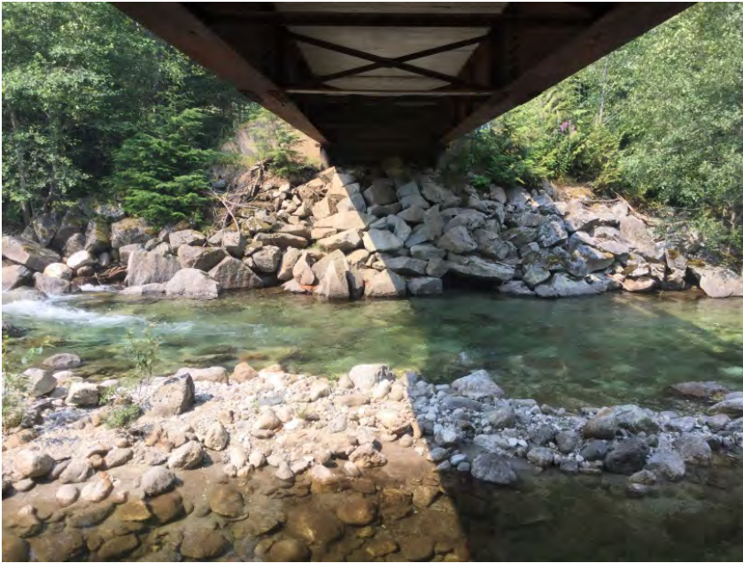
Left Bank Abutment when facing downstream
