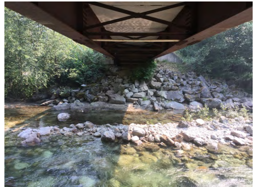
Right Bank Abutment when facing downstream
